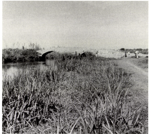
Fig. 62. The bridge at 'Arab al-Milk.
